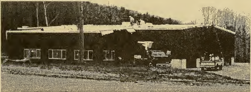
Garage nearing completion of the close in
